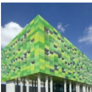
INFRAX WEST TORHOUT
