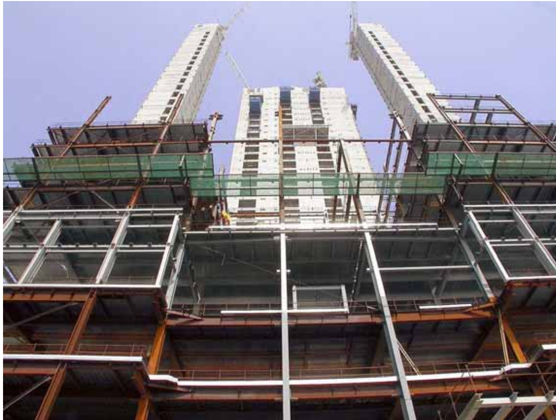
Canary Wharf Building BP1 Cranes on top of Cores
