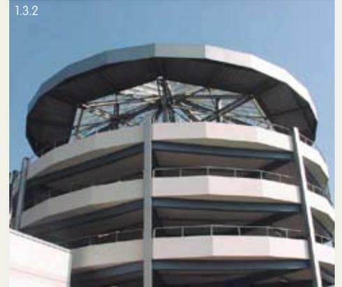
When designing the façade of a multi-storey car park, a major part of the outside walls should remain open (pic. 1.3.2).
