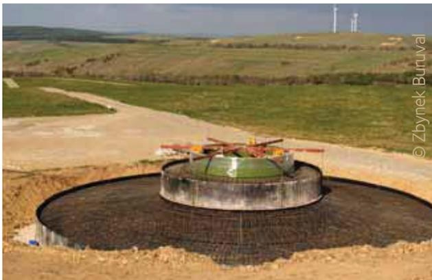
figure 2: Rebars for on-shore foundations
