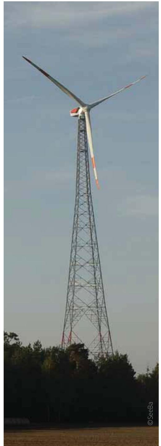
figure 4: Laasow 160 m wind turbine (Fuhrländer)
