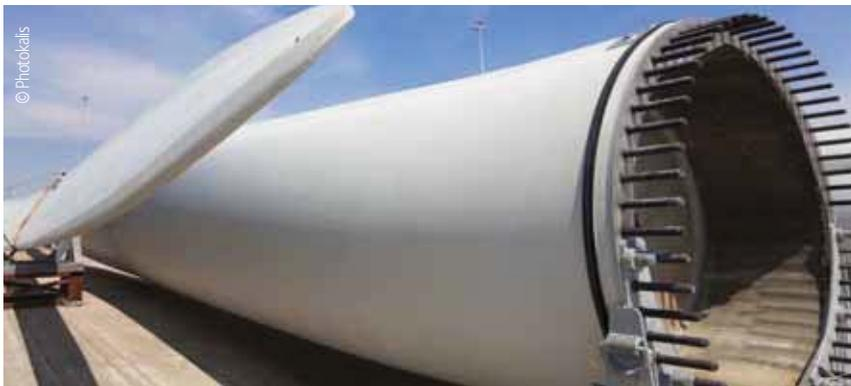
figure 10: Connection for wings
