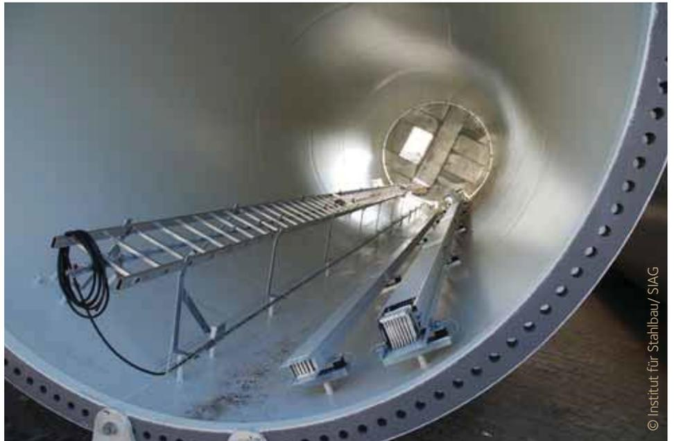
figure 7: Inner part of a tower.
