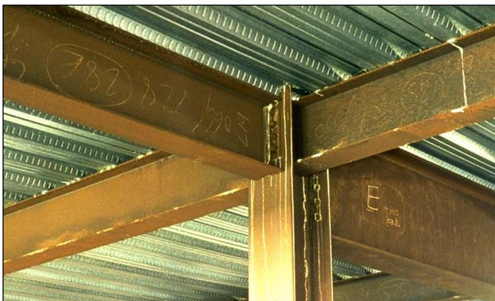
**Figure 1–2 View of unprotected steel structure**
