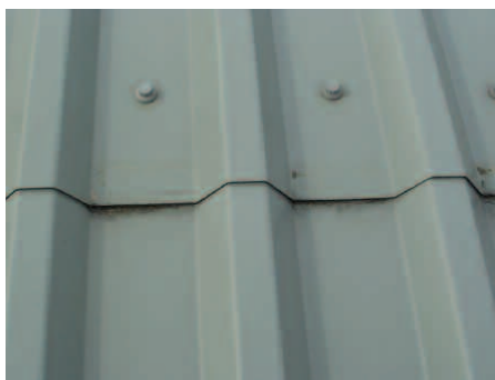
Figure 6. Galvalloy® and Hot Dip Galvanised comparison
